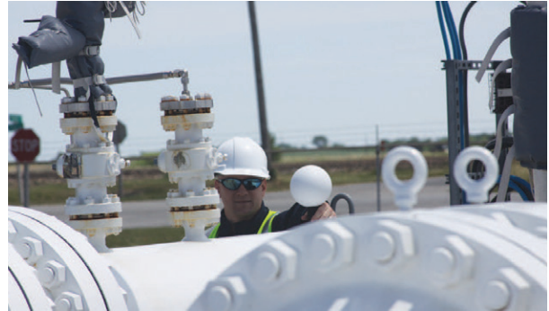
Figure 3: Multiple scans are "stitched" together to generate a contiguous data set. Because of line-of-sight constraints, sites are captured in multiple scans. Scans are then stitched together via a registration process to produce a single contiguous "point cloud." Registration is achieved by establishing common control points via "registration spheres" that are temporarily deployed across the scan site.
